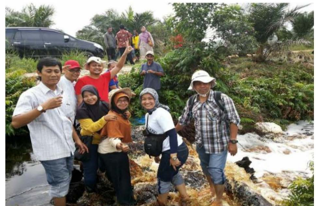
Fig 3. STBA Team is working together, blocking a tributary, wetting peat land area to avoid fire.
